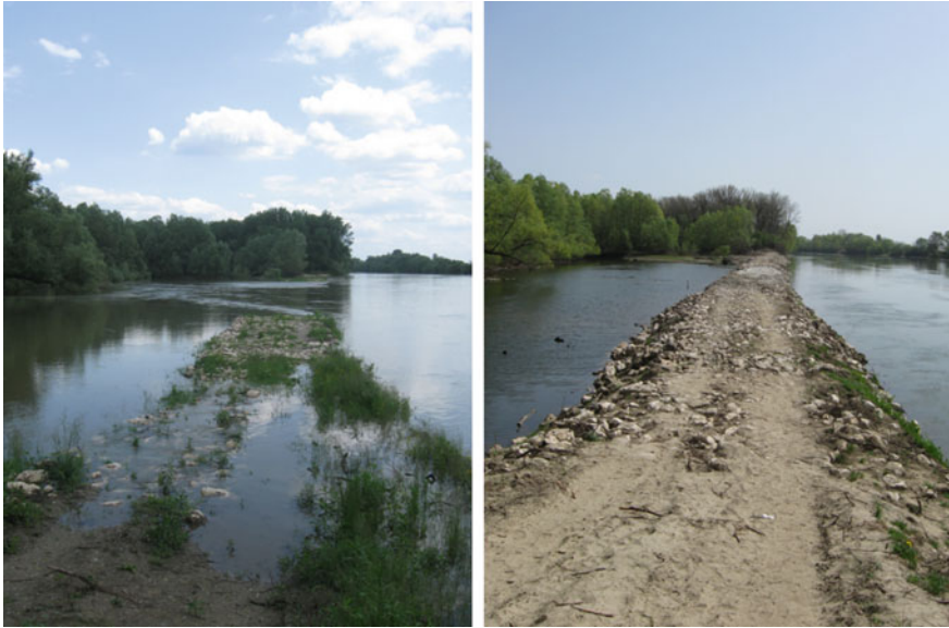
Fig. 20.7 The lowered closure at high and low water stages (photo by Tibor Parrag)
