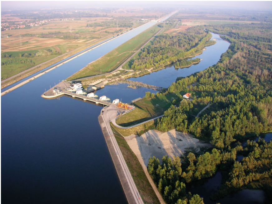
Fig. 9.1 The Dubrava dam with the canal which provides water to the Dubrava HEPP power house and the old Drava channel
