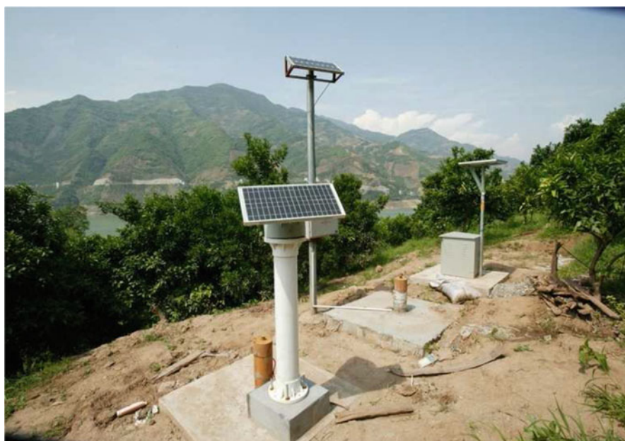
Fig. 3.6 Detecting landslide thrust and groundwater level
