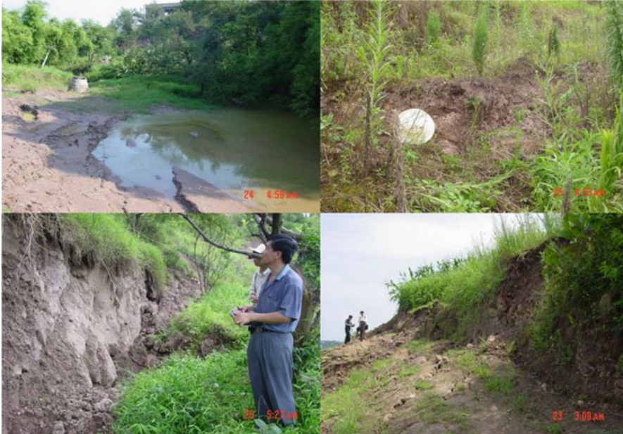
Fig. 3.8 Penetration at the trailing edge of the landslide (the upper-left figure), crack at the trailing edge of the landslide (the upper-right figure), the steep surface between the failed body and the terrain (the lower-left figure), and road deformation in the front edge of the landslide (the lower-right figure)
