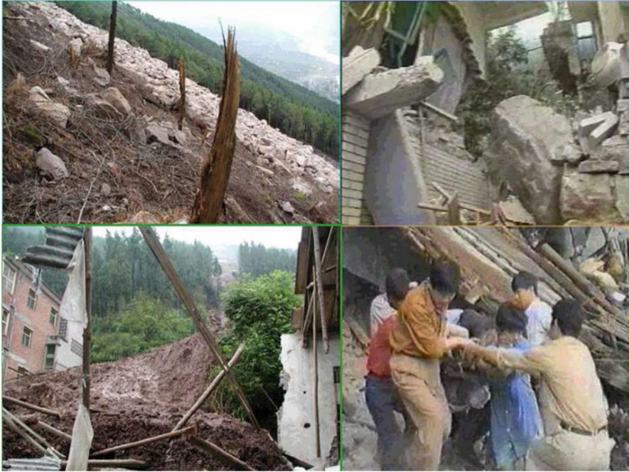
Fig. 3.1 Damages caused by landslides in the Three Gorges area
