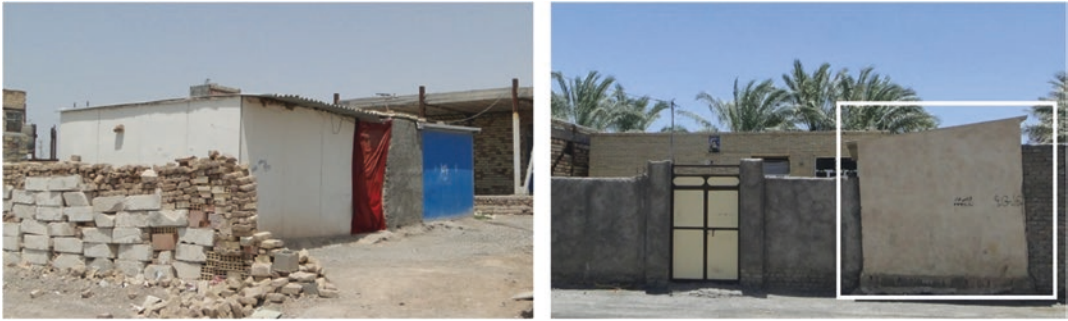
Fig. 3 Prefabricated temporary units (left). Temporary units made of masonry materials (right) (Source: author 2014)
