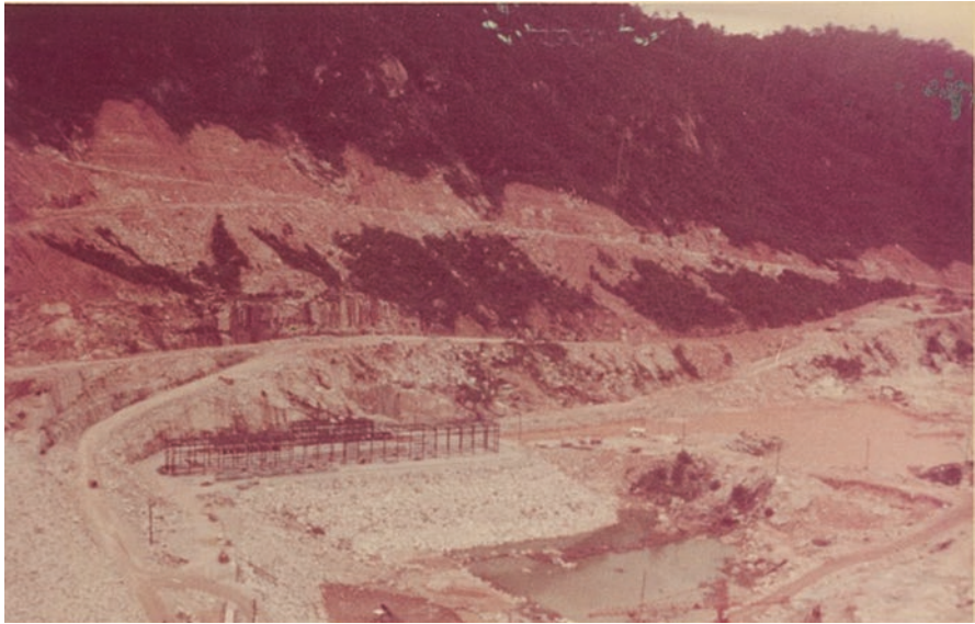
Construction of Sultan Mahmud Dam in 1984 (Photograph by Ab Wahab)
