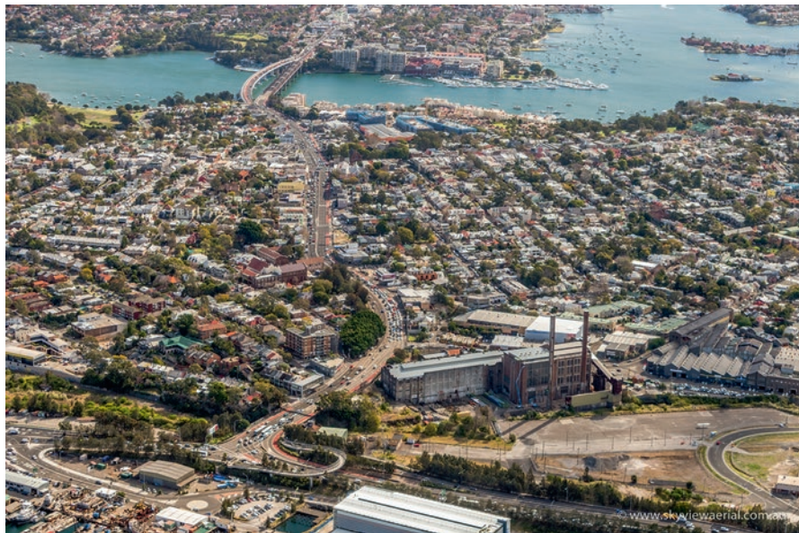
Fig. 5.3 White Bay Power Station. (image: Skyview)
