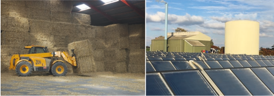
Fig. 9.2 Straw bales for the southern heat grid (left) and solar heat collectors, wood-chip furnace and hot water storage (right) for the northern heat grid of Samsø. (Photos by the author)
