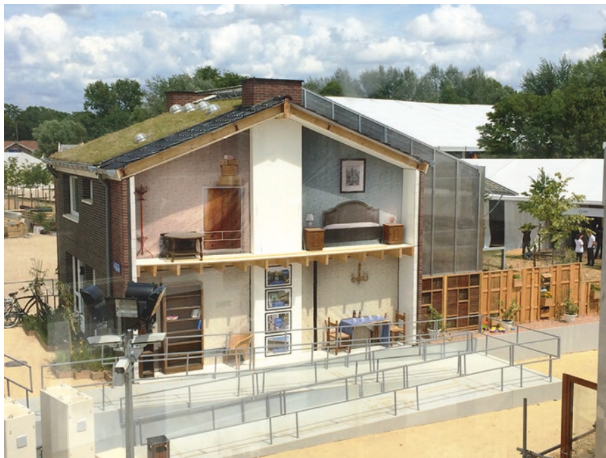
Fig. 9.11 The Prêt-à-Loger house at the Solar Decathlon Europe 2014 competition in Versailles, France. (Photo by the author)
