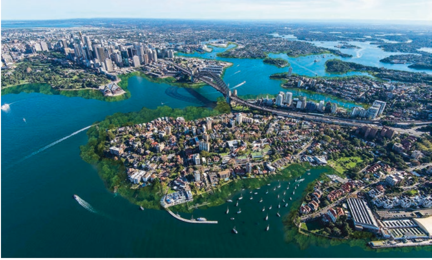
Fig. 9.19 Students' impression of the Sydney sea banks with flood-protective mangrove forest (Image: Jelena Alavanja, Zero Carbon Sydney team, led by Rob Roggema, UTS)
