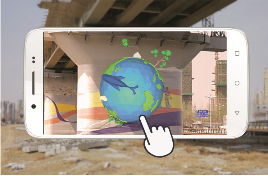
Fig. 2. Yantai Economic Development Area bridge pier 122.
