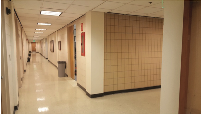
Fig. 7. Image of the hallway where indoor laser scan experiment was carried out
