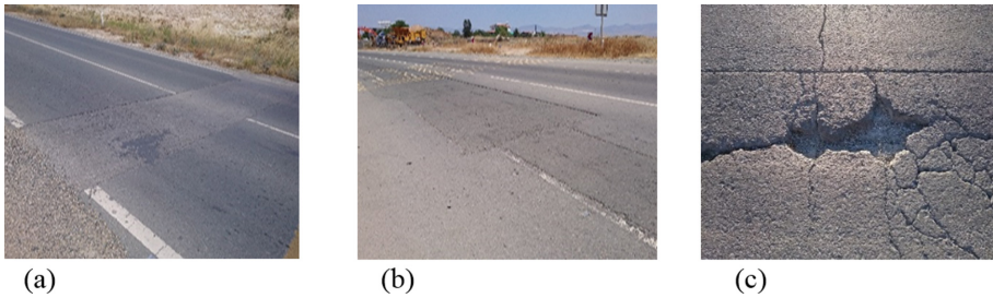
Fig. 1. Pavement surface anomaly types examined for detection and classification: (a) transverse defect/anomaly; (b) longitudinal defect/anomaly; (c) potholes/manholes.
