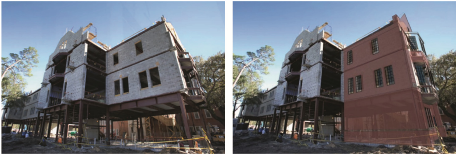
Fig. 5. Completed BIM model augmentation over on-site construction progress documentation
