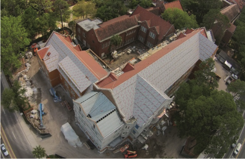
Fig. 13. Construction progress image captured via an UAS.
