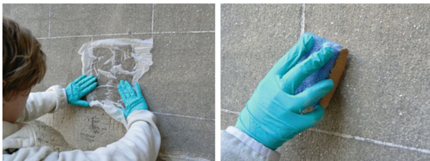
Fig. 6 Two appropriate cleaning methods: Mora cleaning gel covered with Japanese paper [left] and scrubbing with a dry Wishab sponge [right] (Source Govaerts 2012)
