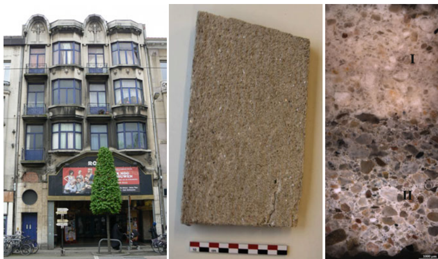
Fig. 1 Historic cinema “De Roma” (1928, north façade), Antwerp (Belgium): upper floors are finished with Terranova (Picture: Y. Govaerts) [left]; Terranova sample from the west façade of “De Roma” (Picture: L. Dekeyser) [middle]; Optical microscopic image of the layered structure of the historic sample: I. Top layer, II. Rendering layer (KIK-IRPA 2011) [right]
