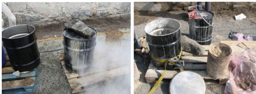
Fig. 9 Lime slaking under pressure in an oil drum
