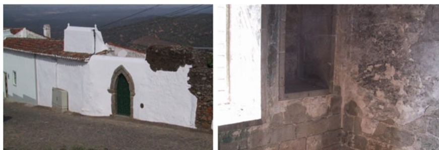
Fig. 1 Whitewashed façade at Terena village, Alentejo, south Portugal (on the left) and a thicker lime coating on stone masonry at Rendufe Monastery, Braga, north Portugal (on the right)
