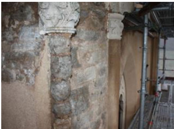
Fig. 3 Stone columns covered with an ochre run-in situ mortar
