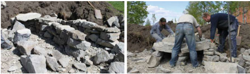
Fig. 7 Field kiln built in 2011. It has two fire places, like some of the kilns found in the region had
