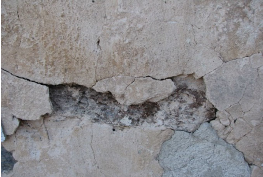
Fig. 4 Old lime mortars in Oviken. The oldest mortars from 17th century are extremely lime rich (20:1 lime/sand by volume) with a yellowish color. What occurs as sand particles to us might be just impurities from the limestone and the slaking process (Balksten and Lindqvist 2016). To reproduce such mortars we need to experiment more with slaking and storing of the specific lime. The surface has traces of lime wash and aging
