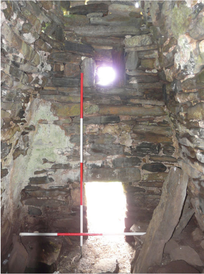
Fig. 2 Corbelled eastern cell, facing west, displaying large patches of multi-layered lime coating. Scale 500 mm ( Photograph M. Thacker )
