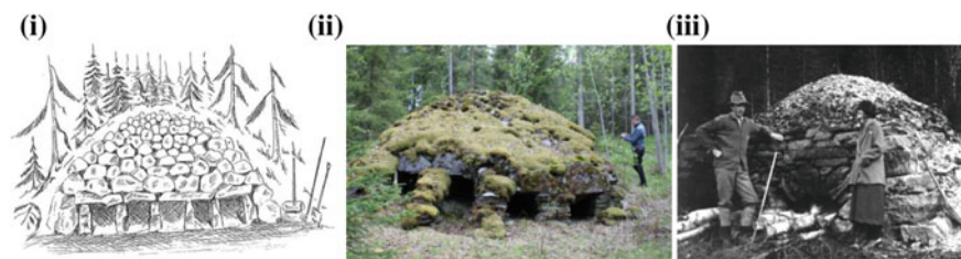
Fig. 2 i Illustration of a field kiln of Jämtland model (Åsling 2000). ii Unburned field kiln built in the late 19th century still standing in the forests of Åse. Now it is covered with moss but originally the stones were visible and not covered. iii Lime kiln from Havsnäs Jämtland in the 1920s
