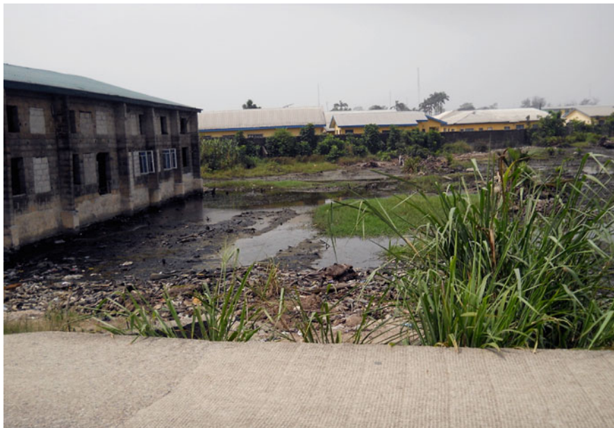
Fig. 13.7 Building of houses right in the mangrove swamp destroys the native mangrove species and open the way for the invasion of the coastal area by alien species such as nypa palms and a variety of grass species. This location was formerly exclusively occupied by mangrove species, but now only a little patch of mangrove stand still remains at the background of the picture. One of the contributing factors is the use of the location as a refuse dump site, which changes the soil to dirty brown that is mixed with greenish algae (e.g. spirogyra ). (Credit: A.O. Numbere)
