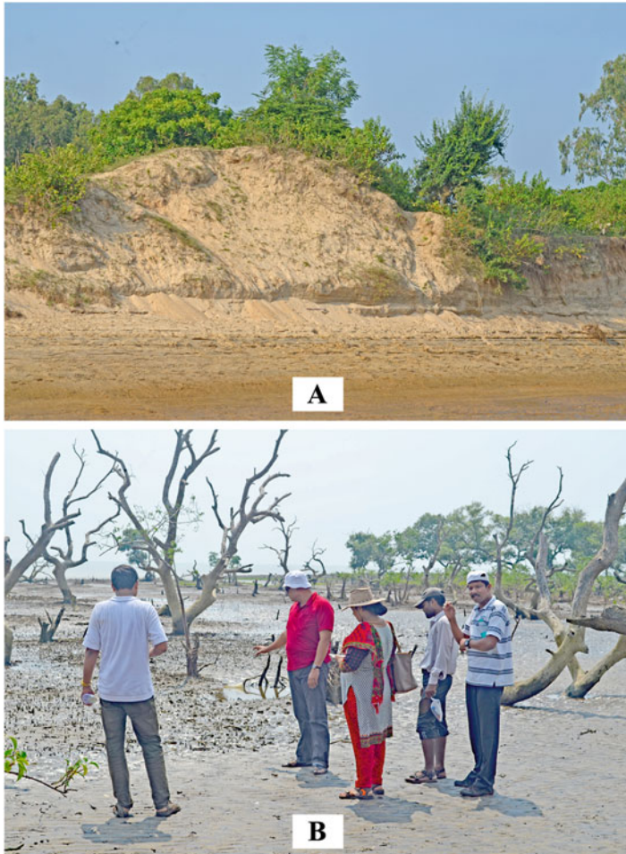
Fig. 6.10 Construction of Hotels Violating regulation of Government of India on Coastal regulatory zone—(a) At Mandarmoni of Midnapore (East) Coast destabilizing Dunes; (b) At Jharkhali of Sundarbans clearing mangroves
