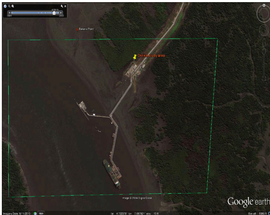
Fig. 13.4 Google image of a major crude oil pipeline linking the Port Harcourt refinery and the sea jetty at Okrika, where crude oil is evacuated and transported abroad. Some years ago (i.e. in the year 2010) this location was exclusively a mangrove forest, but of recent most of the mangrove stands had been taken over by the palms. This is because of constant hydrocarbon pollution from broken pipes, and deforestation aimed at clearing the path along pipeline routes, which results in the death of mangrove trees. (Credit: Google Earth)
