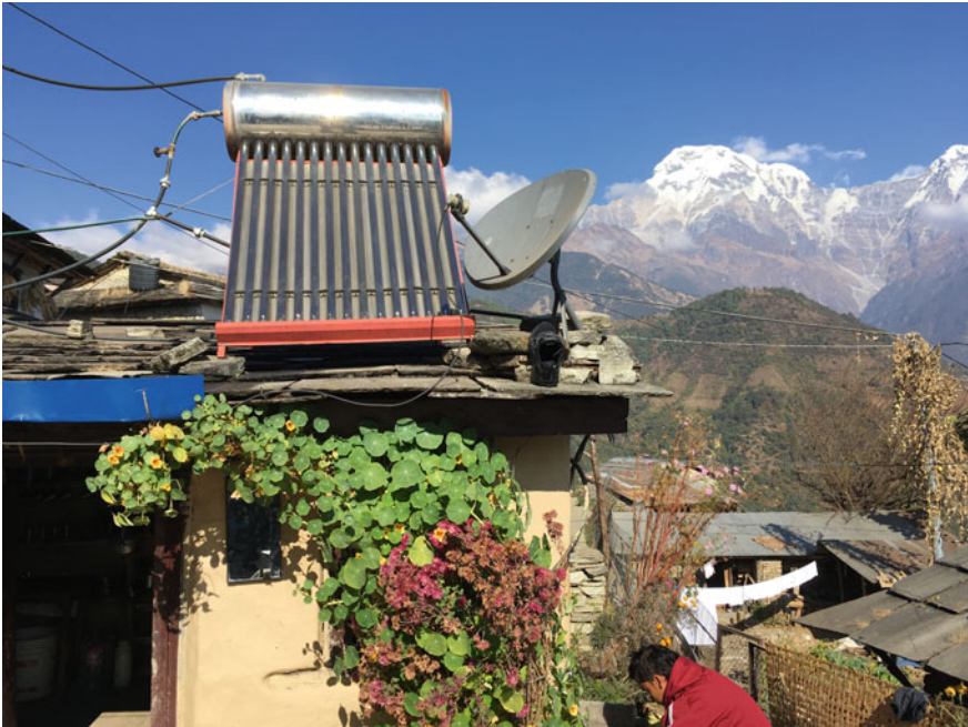
Fig. 1.1 Thermal water heating system
