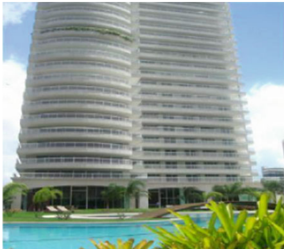
Fig. 24 Examples of building constructions that employ gypsum (building with inner walls in gypsum plaster, São Paulo)
