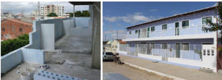
Fig. 22 Examples of building constructions that employ gypsum (flats built in gypsum plaster, in Petrolina and Belem do São Francisco-PE)
