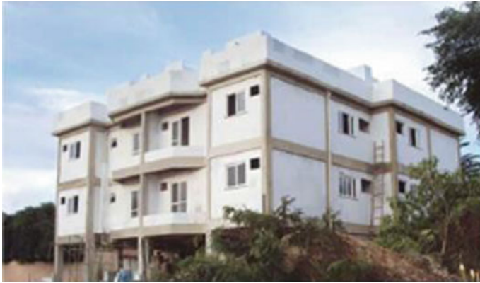
Fig. 25 Examples of building constructions that employ gypsum (building with internal and external walls in gypsum plaster, Rio de Janeiro)
