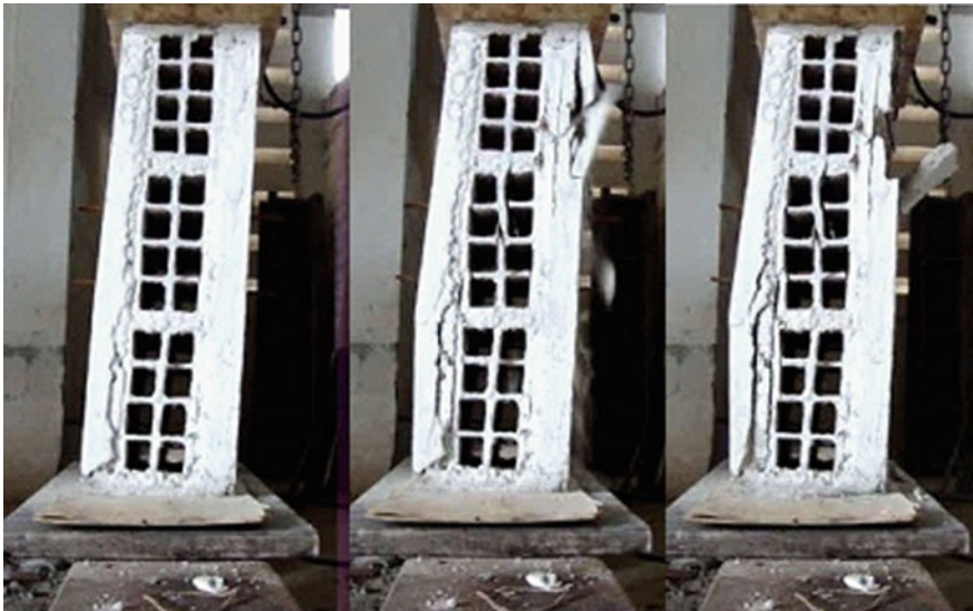
Fig. 16 Rupture of the 3 block prisms with a coating of 1.5 cm and a mix ratio of 1:2:9 reinforced with a POP mesh of 10 \times 10 cm and 4.2 mm of diameter
