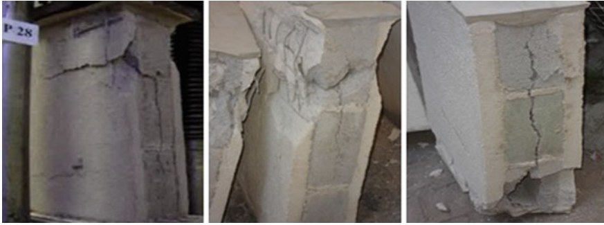
Fig. 14 Rupture of concrete block prisms with coating, steel mesh and connectors
