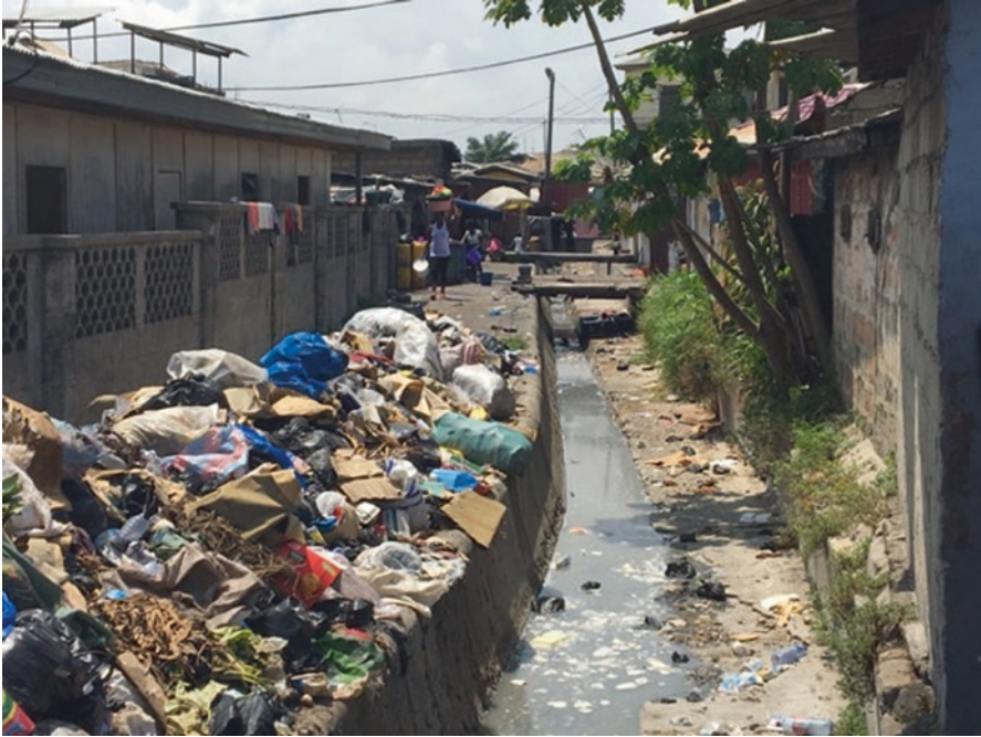
Fig. 3 Drainage ditch clogged with garbage Old Accra, Ghana
