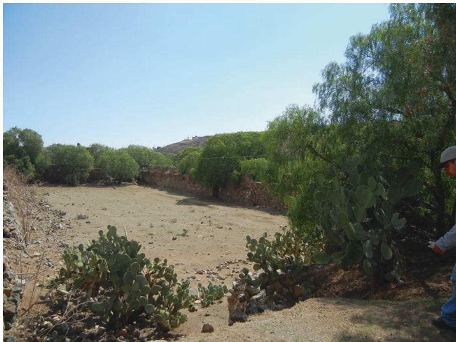
Fig. 5.5 Hacienda de Pánuco, ruins of amalgamation yard and section of the battlemented rampart
