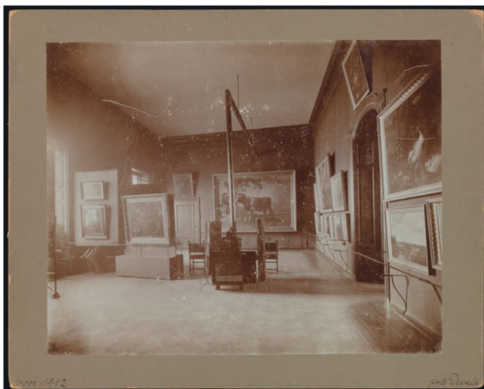
Fig. 16.5 The old museum climate situation: old photograph of the “Potter” Room showing the coal stove in the middle of the room (Mauritshuis archives, with thanks to Q. Buvelot)
