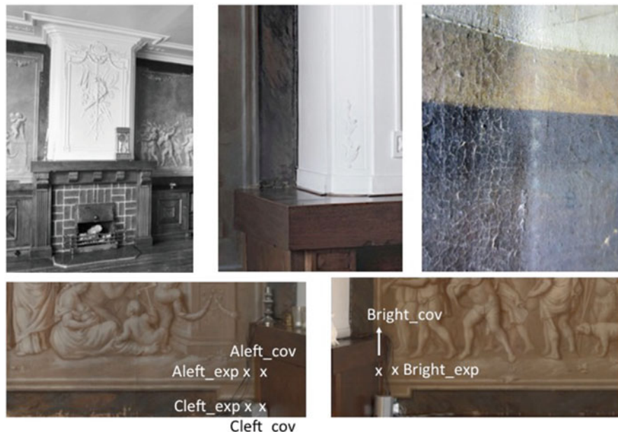
Fig. 6.4 Photograph taken in 1974 of the fireplace with oak panelling on the south wall (photo: RCE) (above left), detail of left side of the panelling covering part of the painting (photo: M.H. van Eikema Hommes, 2013) (above middle) and detail of painting left (east side) to the fireplace, left part is exposed to the room and right part is covered by the panelling (above right) (photo: Keune, 2013). Lower left and right, detail of the paintings left and right to the fireplace with indication of sample areas of A-left_cov, A-left_exp, B-right_cov, B-right_exp, C-left_cov, and C-left_exp
