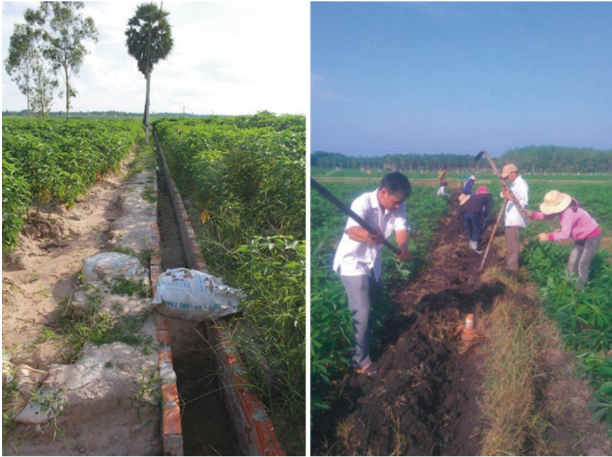
Fig. 16.10 A brick on-farm canal made by farmers (N16-1-10 at Phước Vinh commune), June 2016 (left) and collective work to build an on-farm canal (N 2-22-1-11 at Thanh-Tây commune), March 2017 (right)
