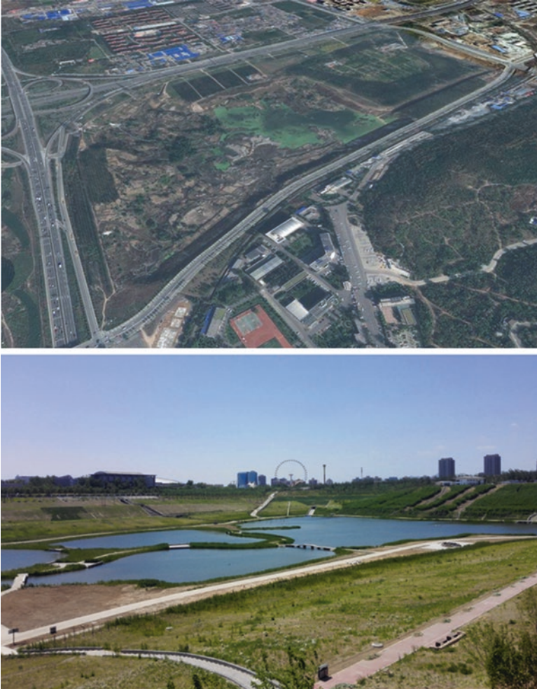
Fig. 3.11 Before-and-after comparison of the West Suburb Sandpit Project
