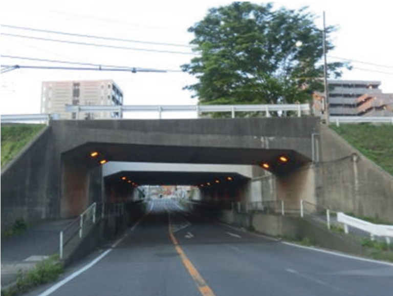
Fig. 4.5 An underpass on the National Road 365, which was flooded in 2013
