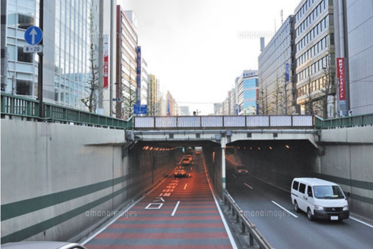
Fig. 4.4 Road underpass where flood inundation depth could be high
