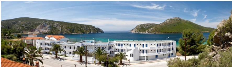
Fig. 59.2 Overall view of the hotel building studied
