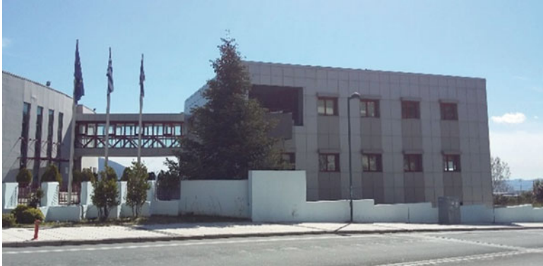
Fig. 60.3 Main facade of Building C
