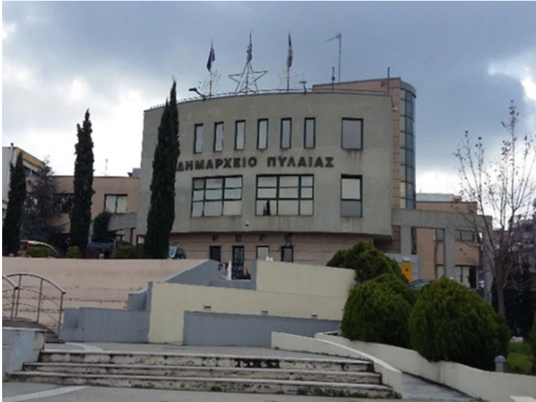
Fig. 60.2 Main facade of Building B
