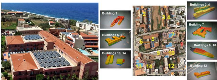
Fig. 52.7 (a) View of hotel roof with installed solar thermal panels, (b) Thermal simulation of hotel buildings
