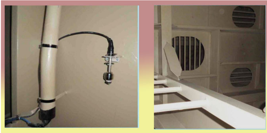
Fig. 8 Termination of the PSPC process in the ballast tanks
