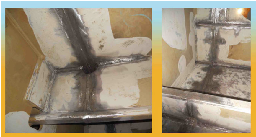
Fig. 7 Secondary surface preparation of affected areas in block's joints
