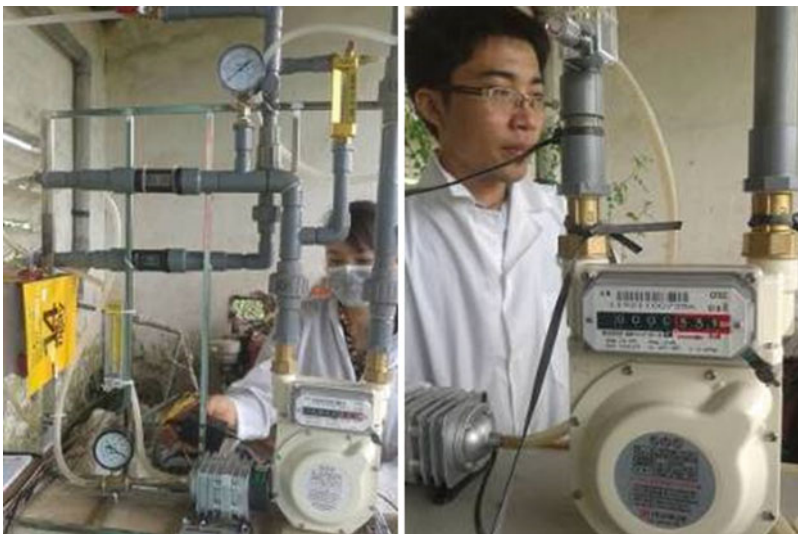
Picture 4 Monitor the biogas flow rate, temperature, moisture, pressure gauge, and biogas volume
