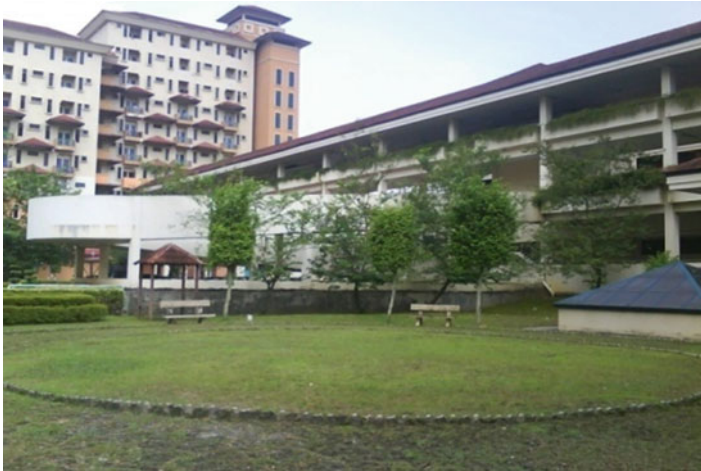
Fig. 4 Allocated site prior to installation (ground level)
