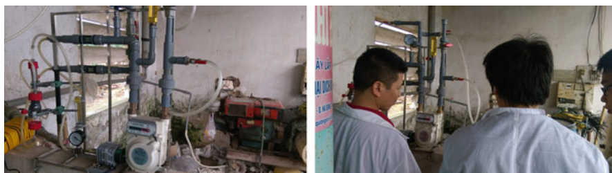
Fig. 4 Pictures of the lab-scale system at Thanh Hung pig farm
