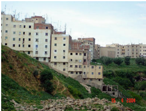
Photograph 1 Constructions in the form of staircases, backed up and raised in height, built on marly lands on steep slopes, near the stream (Oued Fès). They are threatened with collapse due to landslides on these cliffs (Northeast zone of Fez)
