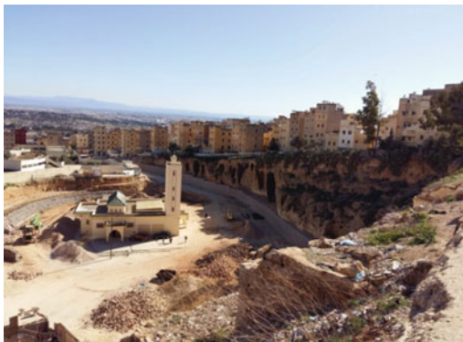
Photograph 2 Chaotic landscape of high-rise constructions that directly joins travertine cliffs a few meters deep. They remain susceptible to collapse (North zone of Fès)
