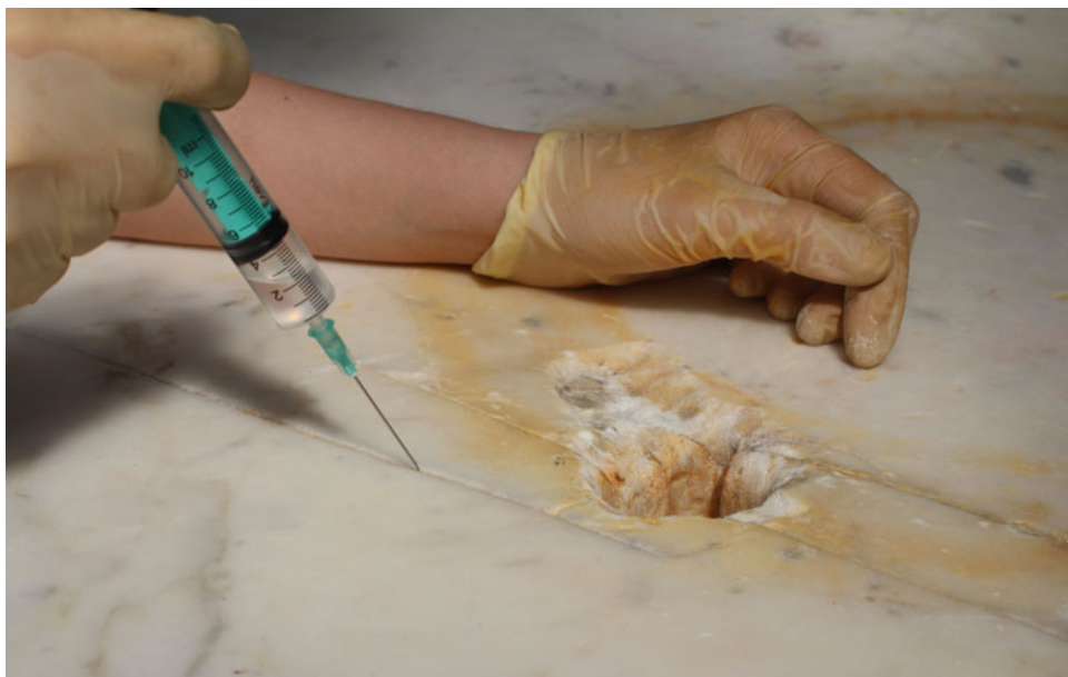
Fig. 5.51 Injection of cracks on the marble with an adhesive compound
