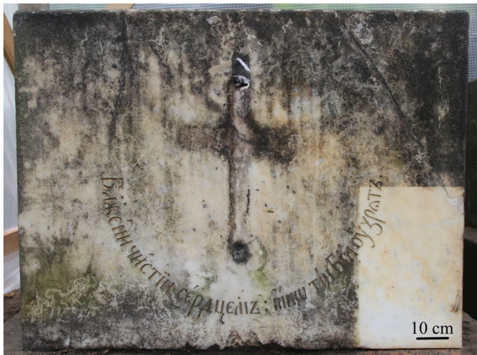
Fig. 5.45 Mud buildups, algae growths, colonies of dark-colored fungi and cracks on the butt end of the marble tombstone of N.M. Karamzin (June 2016, shows the result of trial cleaning)
