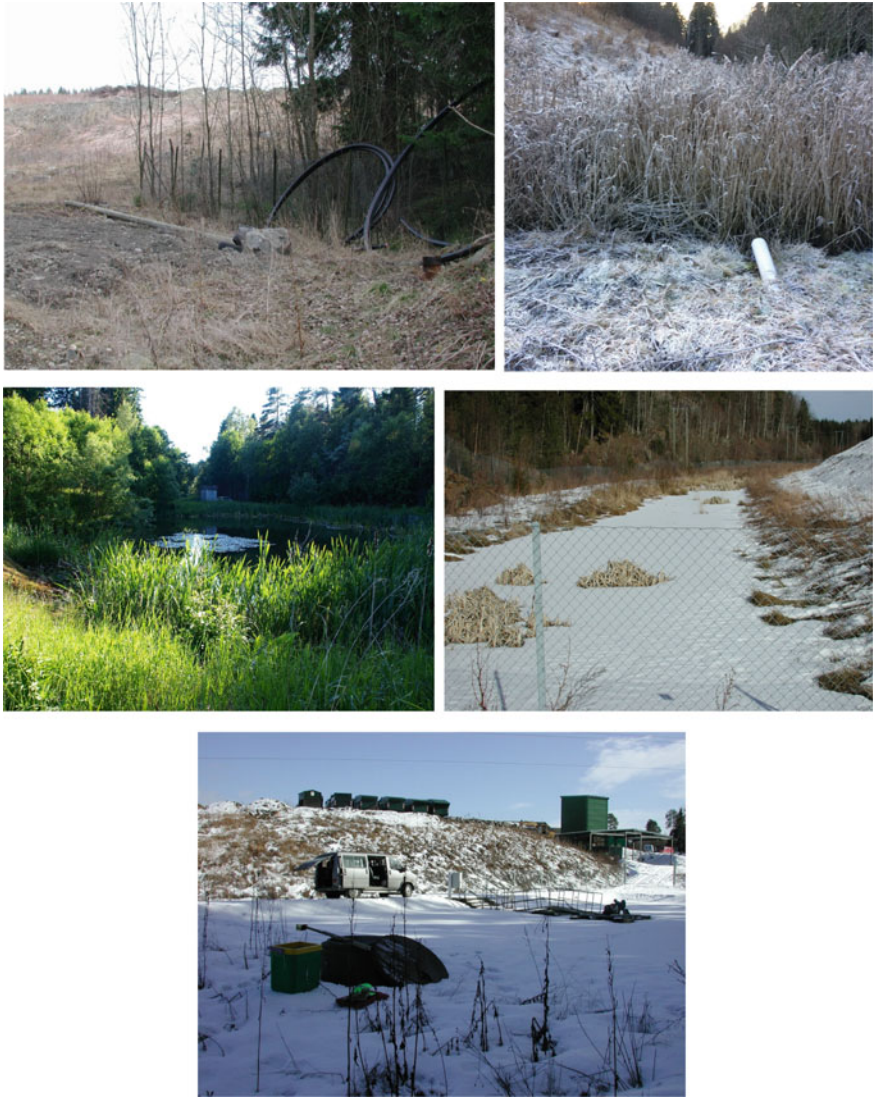
Fig. 13.2 Closed landfill with leachate treatment in wetland. Photograph Haarstad
