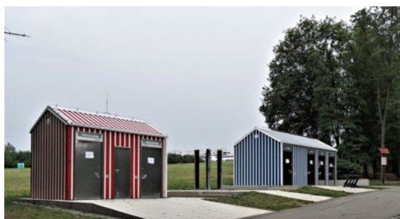
Fig. 1.26 Barrier-free toilets and changing rooms ( Photo Kotásková )
