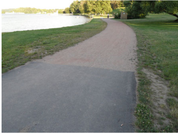
Fig. 1.16 A suitable access road near a water body: the asphalt surface is laid on a base made from mechanically reinforced aggregate which is well compacted ( Photo Kotásková)
