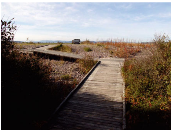
Fig. 1.15 Suitable surface of a corduroy trail for wheelchair users ( Photo Fialová )
