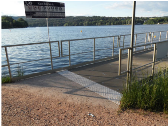
Fig. 1.28 Smooth transition from the boat-stop pier to the path made of mechanically reinforced aggregate ( Photo Kotásková )
