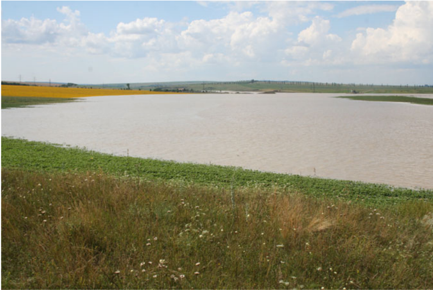
Fig. 6.10 Stanca–Costesti Hydro-Energetical Junction at its peak flooded level during the backwater in the summer of the year 2008. Source Author
