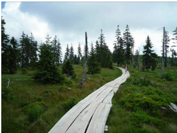
Fig. 1.14 Unsuitable design of a corduroy road ( Photo Kotásková )
