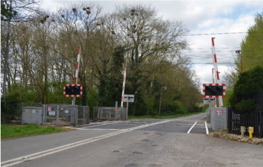
Fig. 1 Carlton level crossing (MCB-CCTV)
