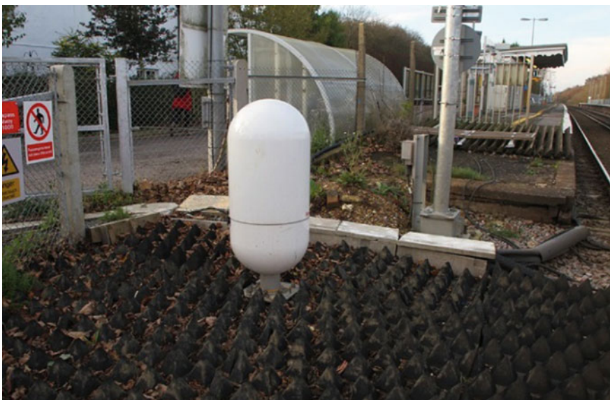
Fig. 11 A radar/LIDAR detector being used at a level crossing in East Sussex (Rail Engineer 2015a, b)
