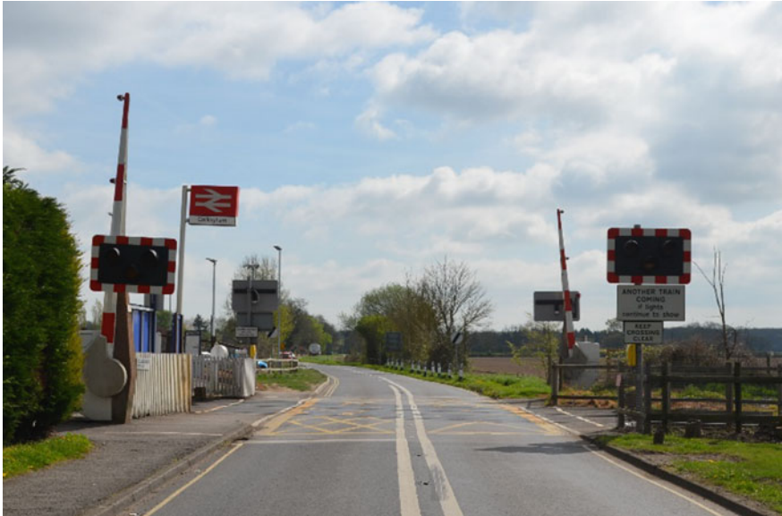
Fig. 2 Collingham level crossing (AHB)
