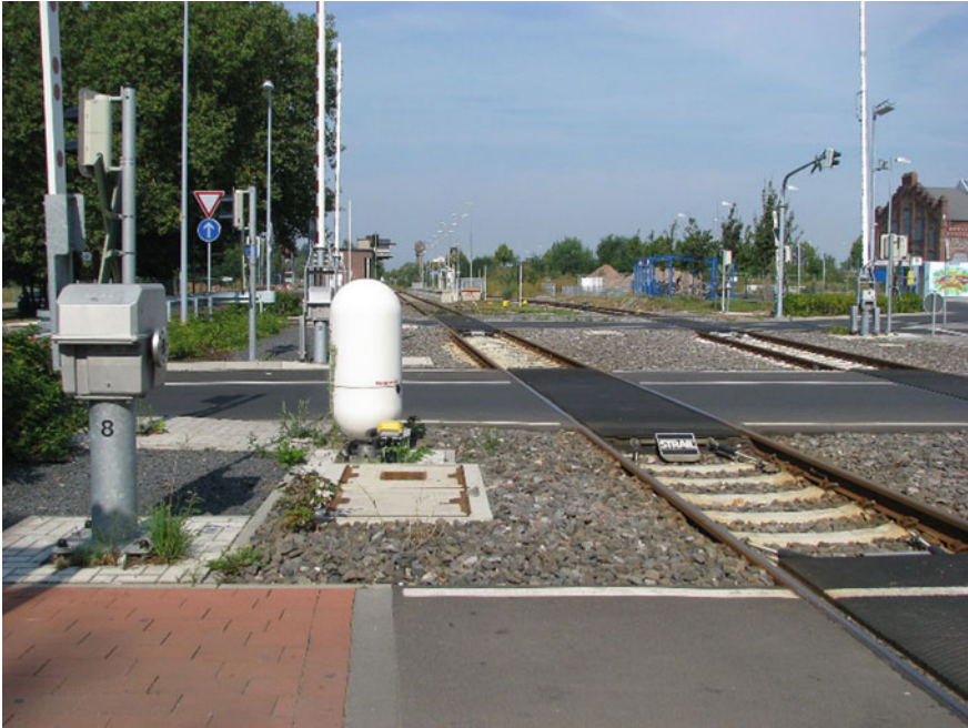
Fig. 13 A radar detector in place at one a German level crossing (ACBahn 2013)
