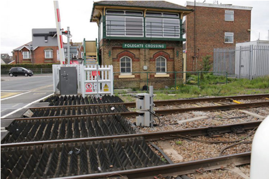
Fig. 15 Polegate crossing, MCB-OD (Rail Engineer 2015a, b)
