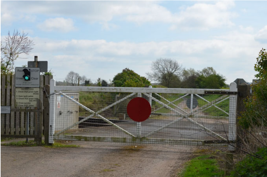
Fig. 4 Westbrook Lane level crossing (UWC-MWL)
