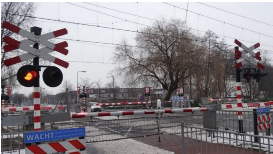
Fig. 14 The Netherlands level crossing with radar detection (UIC 2013)
