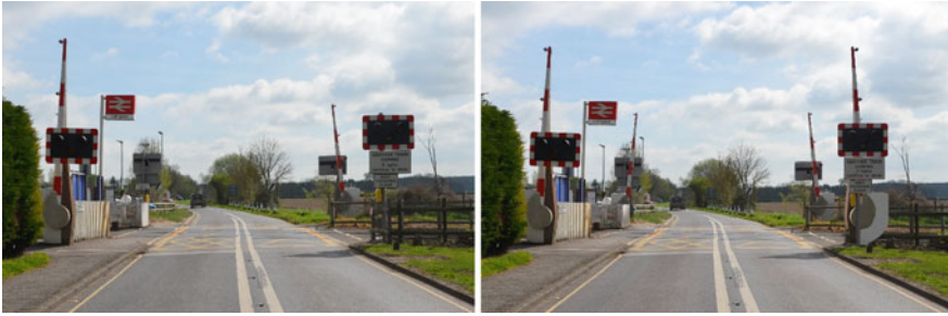
Fig. 17 Left: The current set-up at Collingham level crossing (AHB). Right: Edited image showing barriers on both sides of the road for the introduction of obstacle detection
