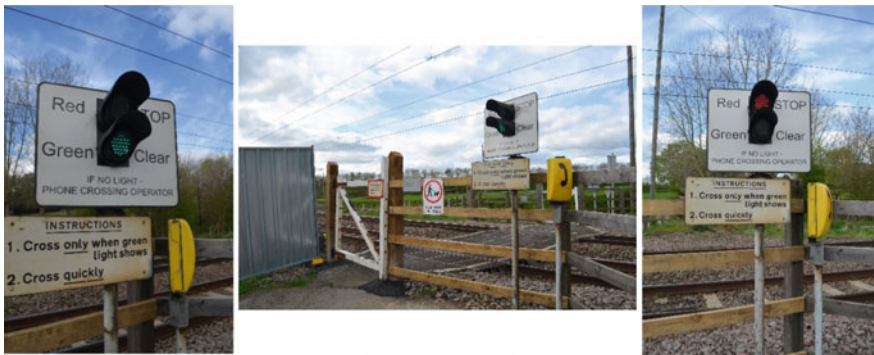
Fig. 3 Eaves Lane level crossing (FP-MWL). From left, miniature warning lights showing it are safe to cross, image of level crossing, miniature warning light showing that a train is approaching and it is unsafe to cross
