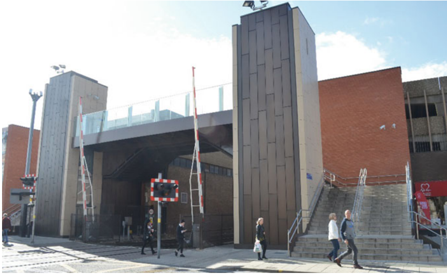
Fig. 7 Footbridge over Lincoln High Street level crossing
