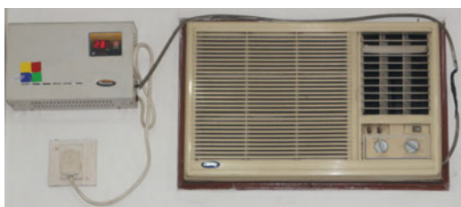
Window air conditioner
