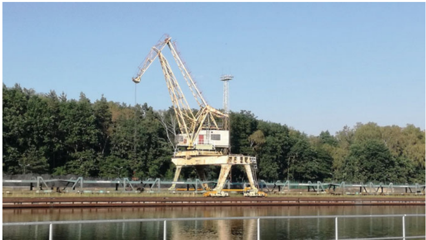
Fig. 10 Jib crane for bulk material handling in the Gliwice logistic centre
