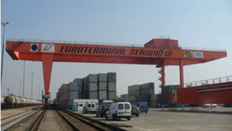
Fig. 14 Main bridge crane for reloading of containers in Euroterminal Sławków logistic centre
