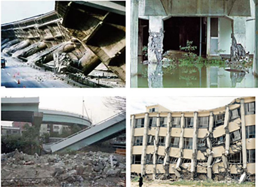
Fig. 43.1 Collapse of bridges and buildings
