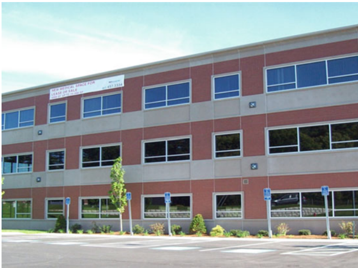
Fig. 1.5 PC cladding on medical building
