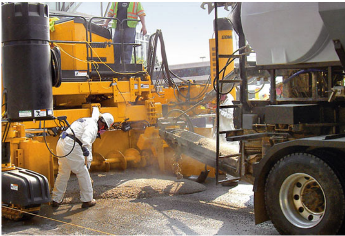
Fig. 35.3 Placement of polyester-styrene PC
