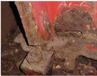
Fig. 95.2 Typical corrosion example of steel bearing
