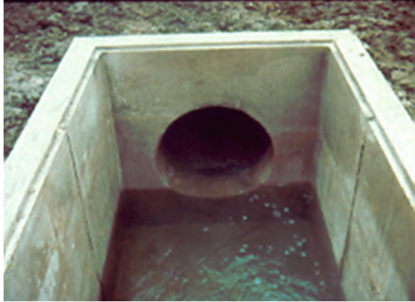
Fig. 1.2 Precast sump for acid waste
