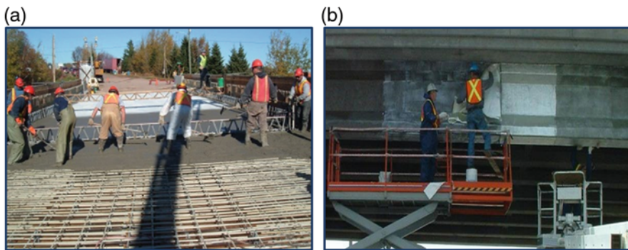
Fig. 5.2 (a) Deck slab reinforced with GFRP. (b) Installation of GFRP sheet
