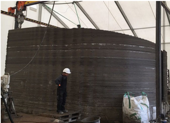
Fig. 1.11 Building placed with 3D printing [9]
