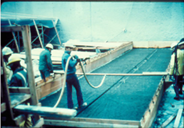
Fig. 39.2 Applying monomer (USACOE) on stilling basin floor
