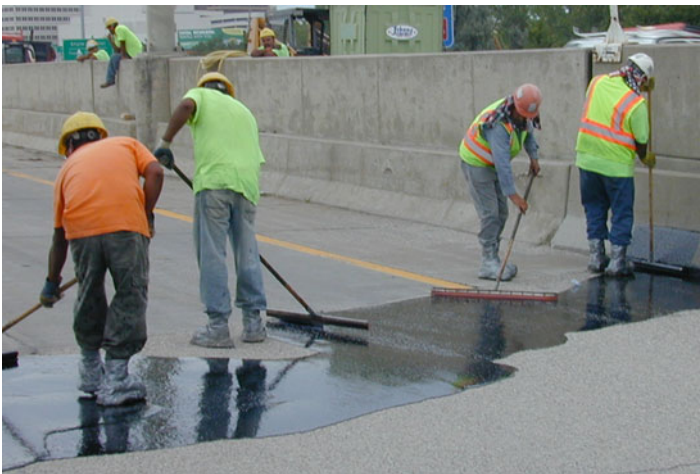
Fig. 35.1 Applying epoxy to clean surface
