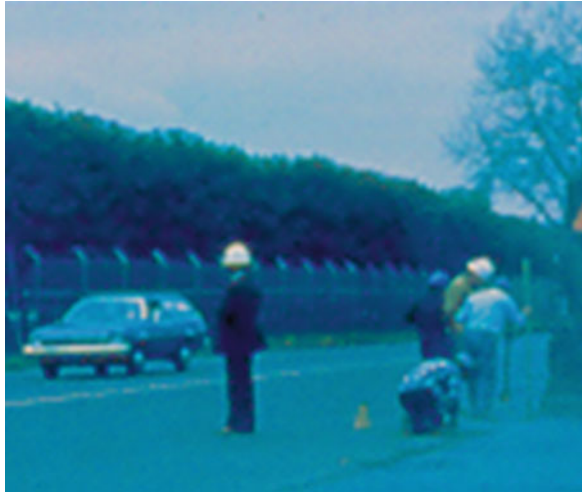
Fig. 1.4 Paving with sulfur concrete
