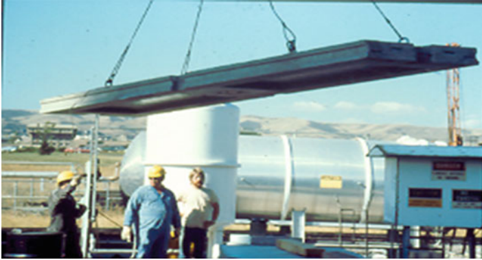
Fig. 39.1 Pretensioned PIC bridge slab (BuRec)
