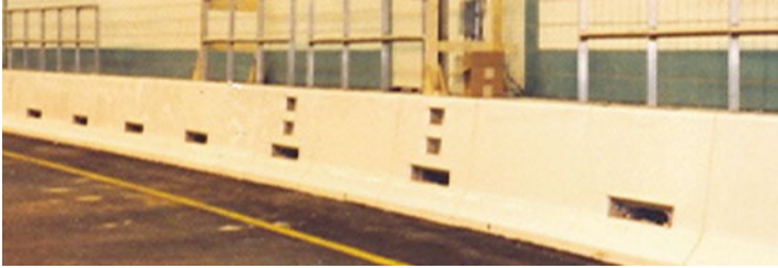
Fig. 44.5 Stair treads and precast blockouts
