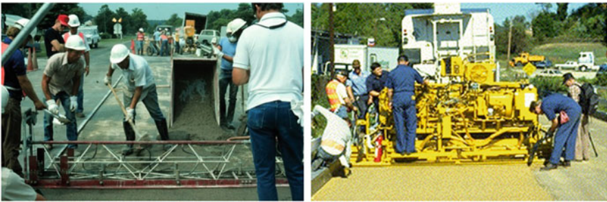
Fig. 2.3 PM polyester concrete placement: vibrating screed is used to consolidate and strike off PC (left); continuous batching and paving are used (right)
