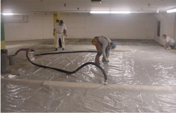
Fig. 39.6 Vacuum impregnation process impregnation
