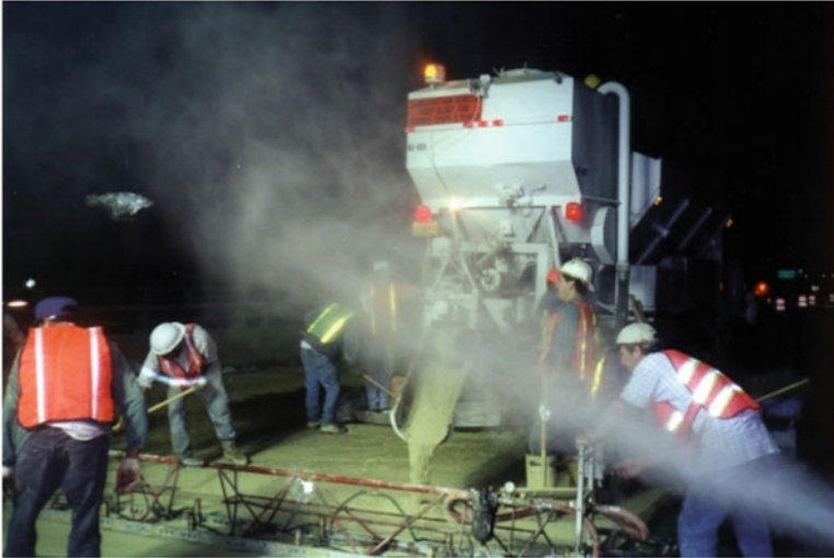
Fig. 2.1 LMC-VE overlay placed at night. Fogging to increase the humidity
