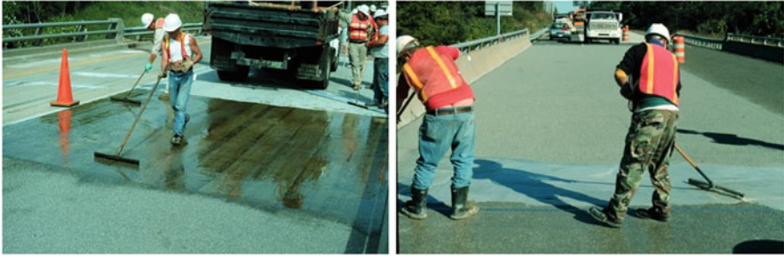
Fig. 2.2 Notched squeegees are used to place ML epoxy overlay (left). Slurry mixed with mortar mixers is struck off with gage rakes (right). Basalt aggregate is broadcast to excess onto both overlays
