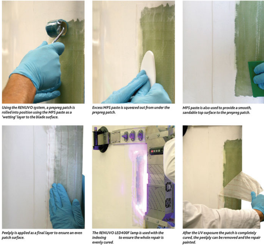
Fig. 8.8 The standard procedure of RENUVO™ system (Marsh 2011)
