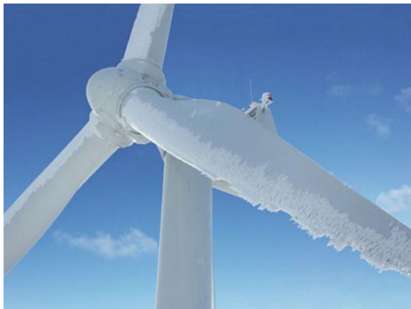
Fig. 12.5 Illustration of icing blades (Muñoz et al. 2016)
