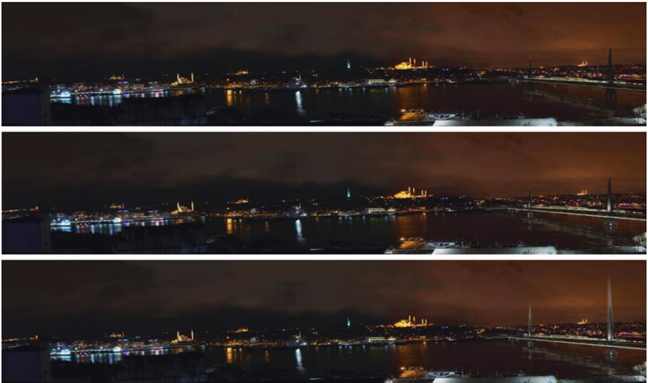
Fig. 73.17 The three possible solutions for the architectural lighting during the night: 1, silent presence (the bridge is illuminated by a thin light line that accompanies the pedestrian path and connects the two banks of the Golden Horn); 2, cultural lighting (the light illuminates the
