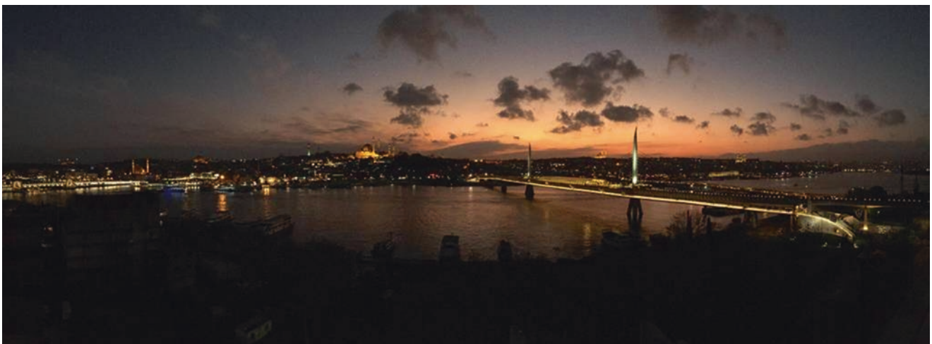
Fig. 73.18 The Haliç Metro Crossing Bridge just after sunset
