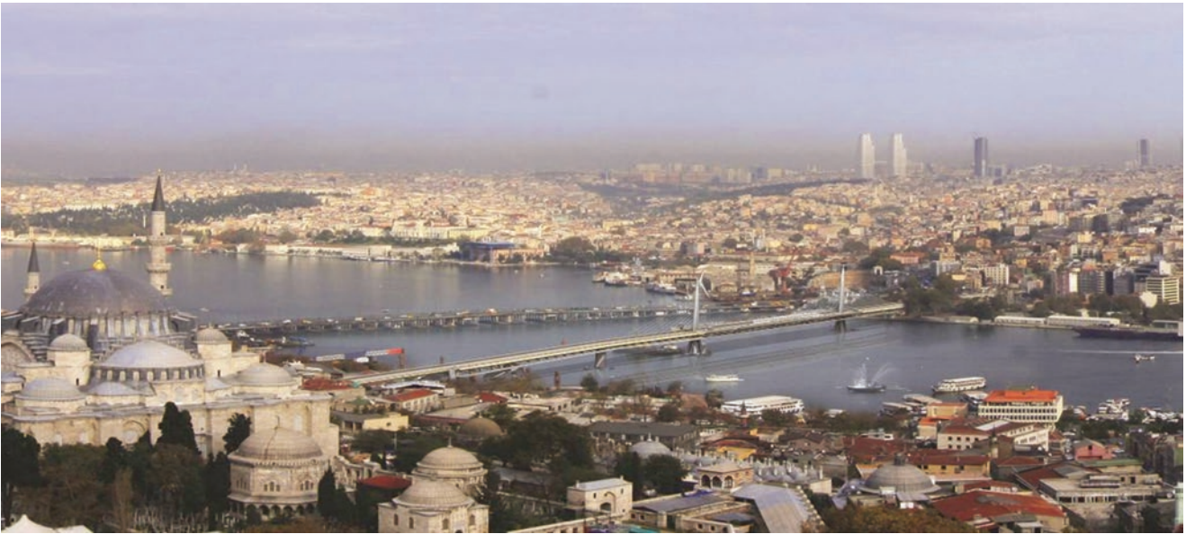
Fig. 73.12 Rendering of the chromatic solution adopted for the bridge. This solution privileges the coherence of the work with the surroundings by choosing a chromatic treatment related to the elements present in the context and weighted according to their meaning
