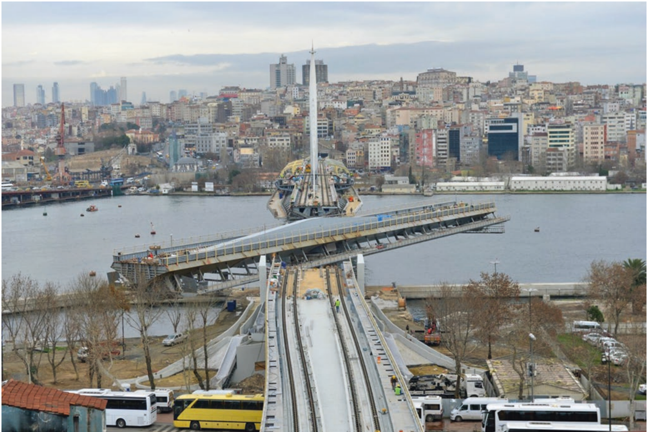
Fig. 73.9 The swimming bridge during the test opening operations
