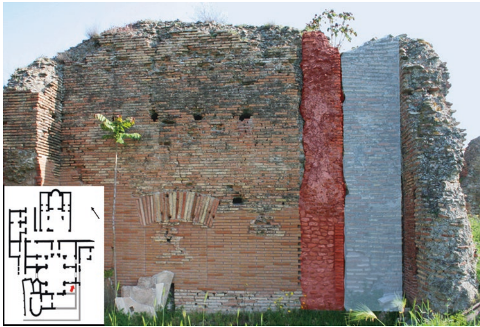
Fig. 52.5 Frigidarium, southeast wall of the quadrangular bath, exterior. The new use to which this sector of the building was put modified the layout of the rooms and transit areas, levelling the masonry flush with the wall on the eastern side in the room next to the bath (in red) and closing the services corridor with a brick infill interspersed with very thick layers of mortar (in grey). The entire surface was then clad with
