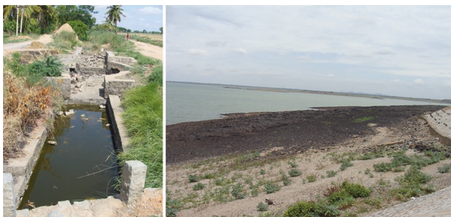
Fig. 1.4 Intensive canal system and water reservoir of river dam are the legacy of the Green Revolution. Current dilapidated irrigation infrastructure and insufficient water in the reservoir due to droughts raise question on sustainability of the Green Revolution
