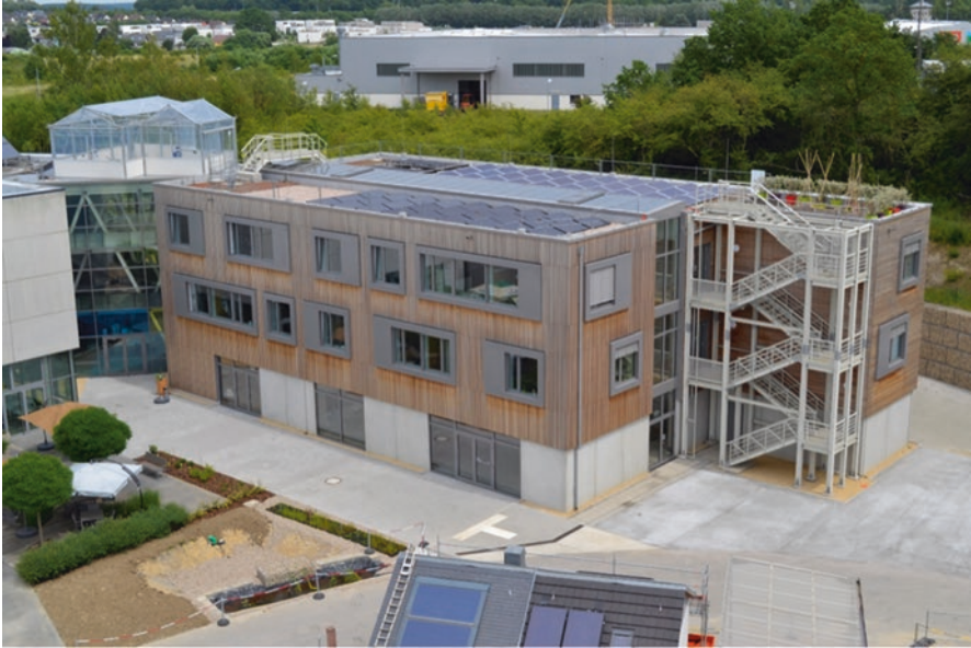
Fig. 8.4 The Neobuild Innovation Centre (Photo courtesy of Neobuild)
