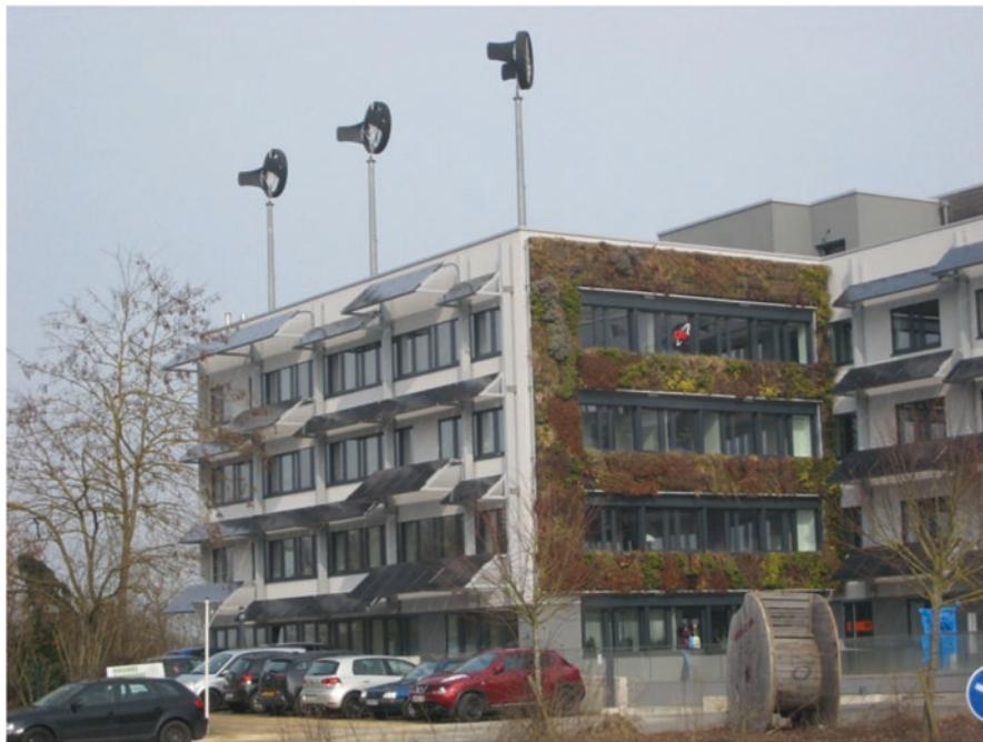
Fig. 8.5 The Solarwind building: green façade, solar panels and roof wind turbines (Photo: Bérénice Preller)
