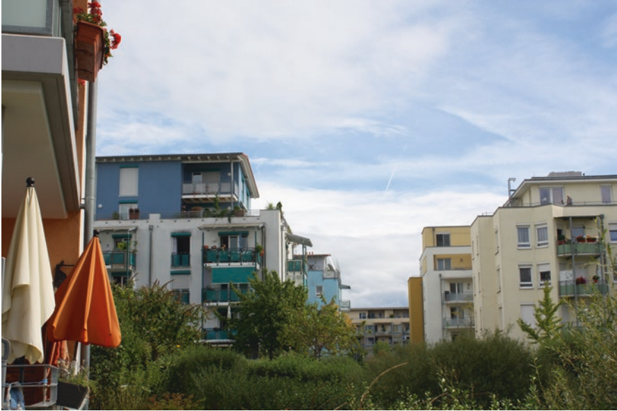
Fig. 5.4 Multifamily housing in Freiburg Rieselfeld (Photo: Sebastian Fastenrath)
