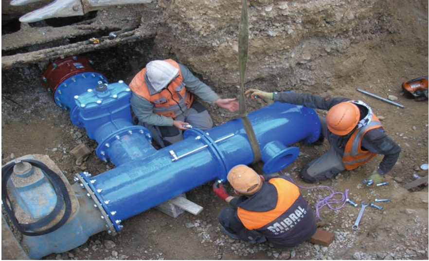
Exhibit 15 Mibral LLC team at construction site; photo © MIBRAL LLC
