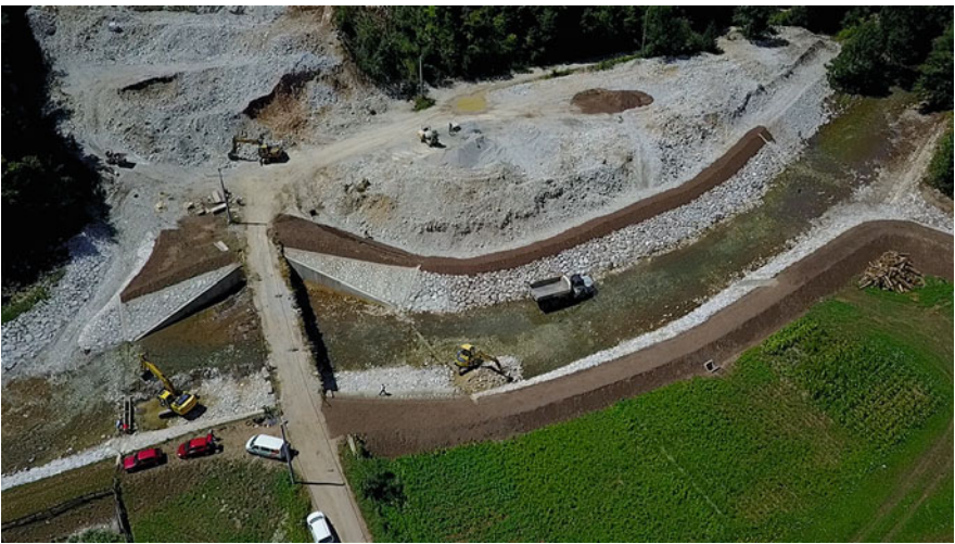
Exhibit 16 MIBRAL LLC at construction site; photo © MIBRAL LLC
