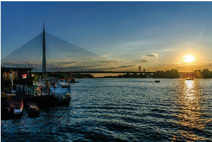
Exhibit 3 Ada Bridge, Belgrade; photo © 2017 Branko Birač
