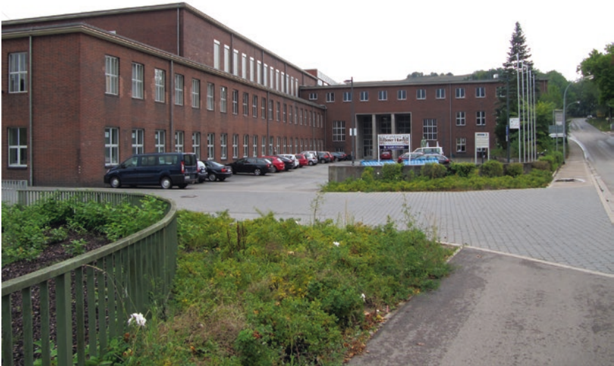
Fig. 46.6 Main building of the former Reden mine, hosting today, among others, the center for Biological Documentation
