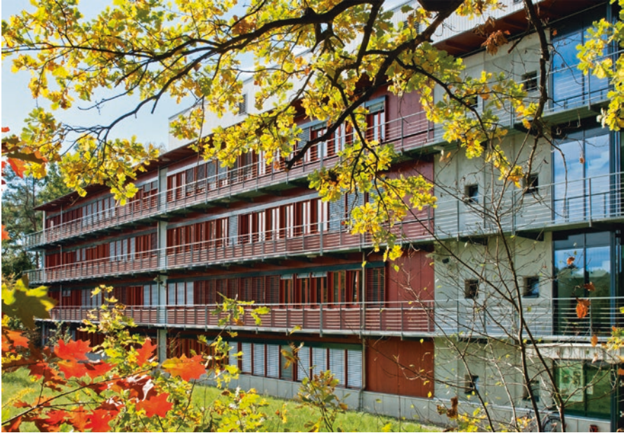
Fig. 21.17 View onto institute building Senckenberg Naturhistorische Sammlungen Dresden, A.-B.-Meyer-Bau in Dresden-Klotzsche, built in 1999 (photo: F. Höhler)
