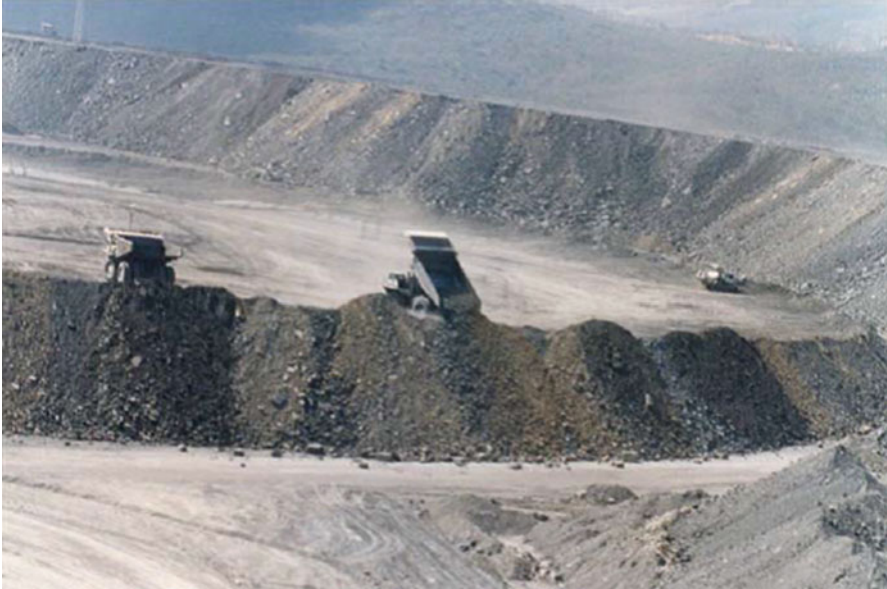
Fig. 2.8 Ending dumping in progress in one of the opencast coal mines [11]
