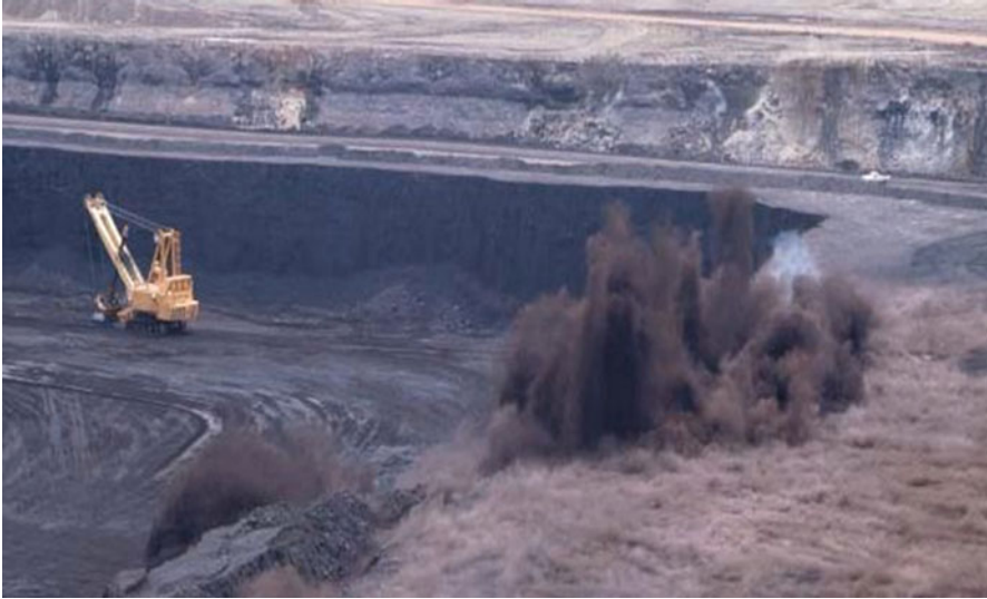
Fig. 2.17 Blast vibrations can cause failures in the dump slopes and hence are designed and analysed accordingly (NCL, India)
