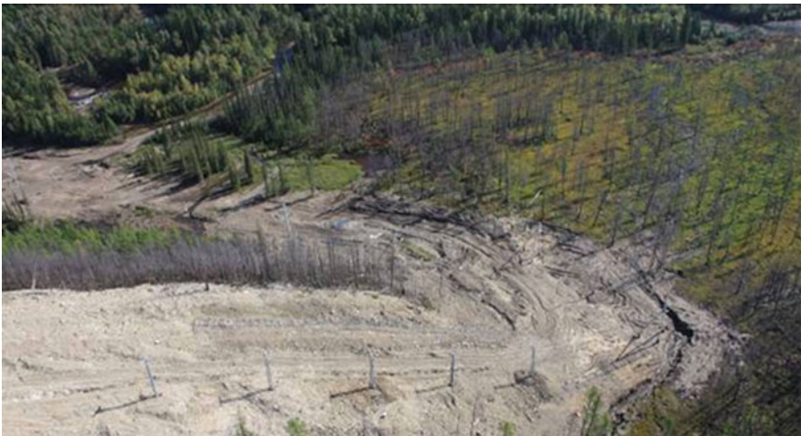
Fig. 14.6 Landslide on a steep slope along pipeline in Chulman area, 2010
