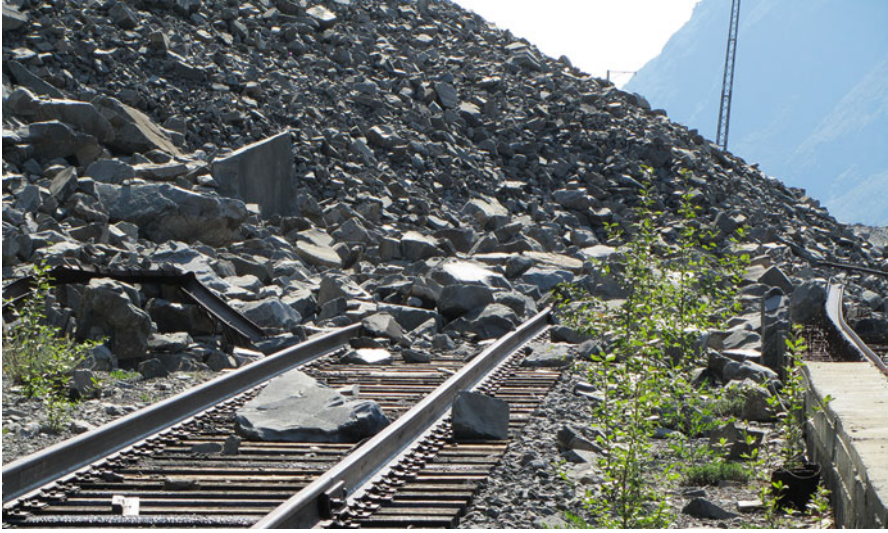
Fig. 14.9 Catastrophic landslide – kurum-shift in the mountain part of Chara-China Railroad, 2015. (Photo by D.O.Sergeev)
