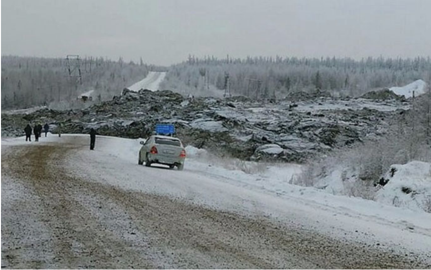
Fig. 14.3 Catastrophic landslide from diamond tailing dump caused by excess pressure in freezing soils near Mimyy. (Photo of November 2015 [2])
