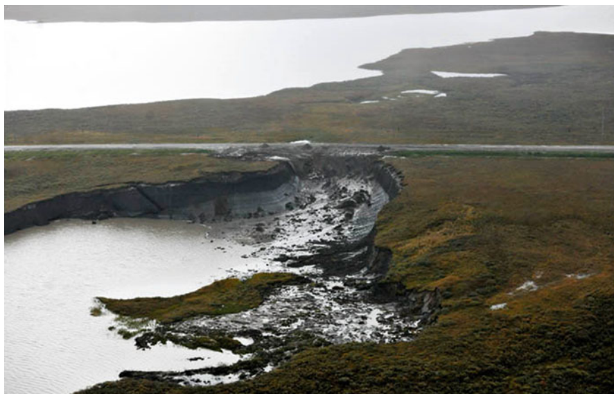
Fig. 14.2 Landslides directed to the road near Bovanenkovo. (Picture of 2016: Vladimir Olenchenko)
