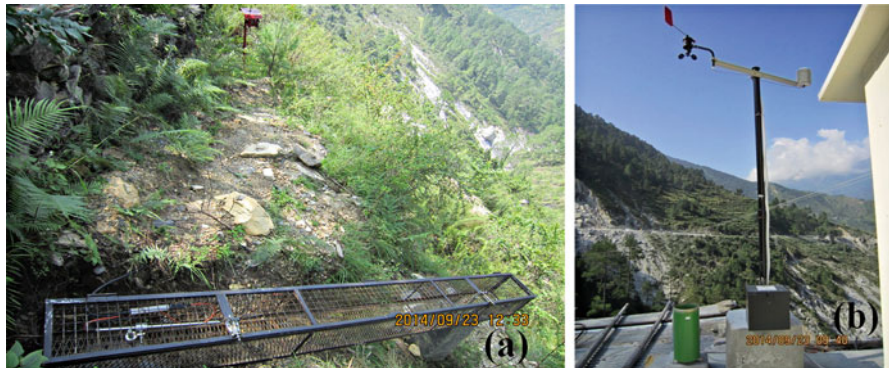
Fig. 6.4 (a) Wire-line extensometer (WLE); (b) Automatic Weather Station (AWS)
