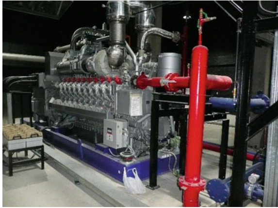
Fig. 3.31 MTU biogas engine installed in power-house solution [MSM Energy Solutions Co., Ltd.]
