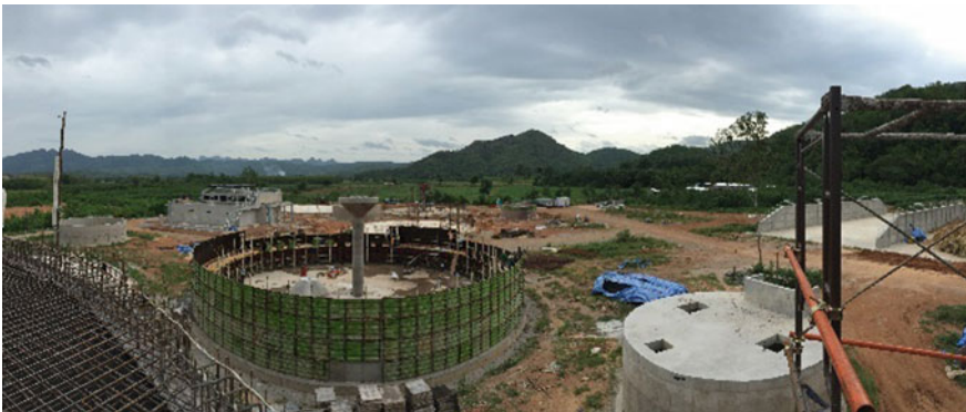
Fig. 3.22 Concrete casted digester during construction
