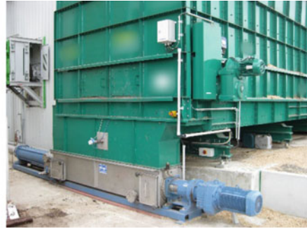
Fig. 3.20 Example of a solid-liquid pump located after the mixing box to send the materials into the digester [Pumpenfabrik Wangen GmbH]
