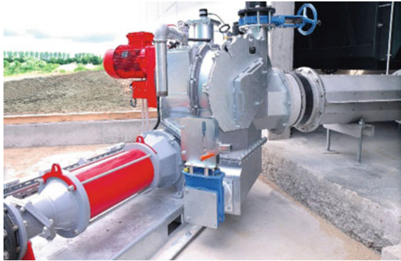
Fig. 3.20 Example of a solid-liquid pump located after the mixing box to send the materials into the digester [Pumpenfabrik Wangen GmbH]
