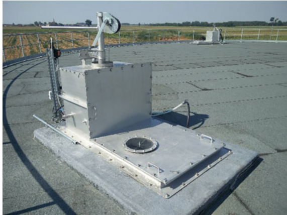
Fig. 3.26 Mixer dome for easy and safe maintenance of submersible mixer in gas tight tanks
