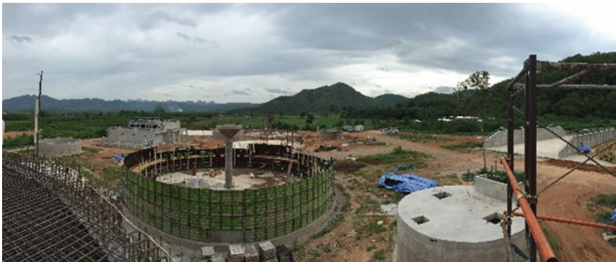
Fig. 3.22 Concrete casted digester during construction
