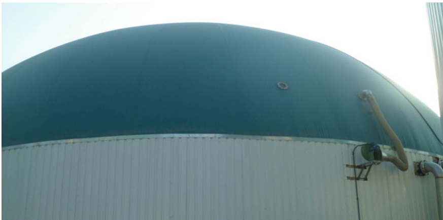
Fig. 8.9 Flexible cover digester
