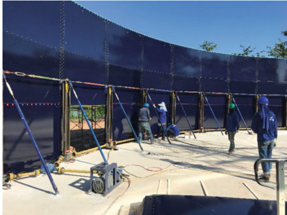
Fig. 3.23 Glass fused tank under installation
