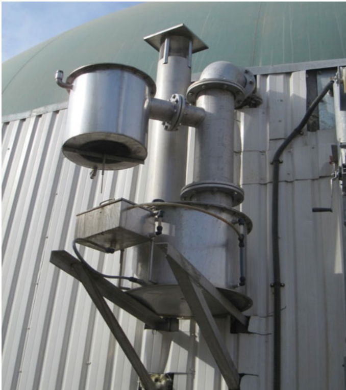
Fig. 8.4 A typical mechanical-based pressure control safety valve
