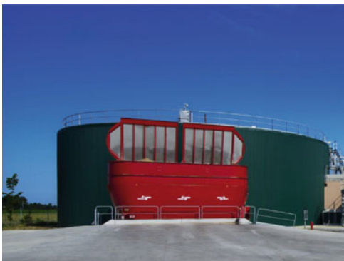
Fig. 3.14 The installation of a vertical mixing screws solid feeder (left) [Sebigas a division of Exergy S.p.A.] and a single vertical screw feeding system (right) [Trioliet B.V.]
