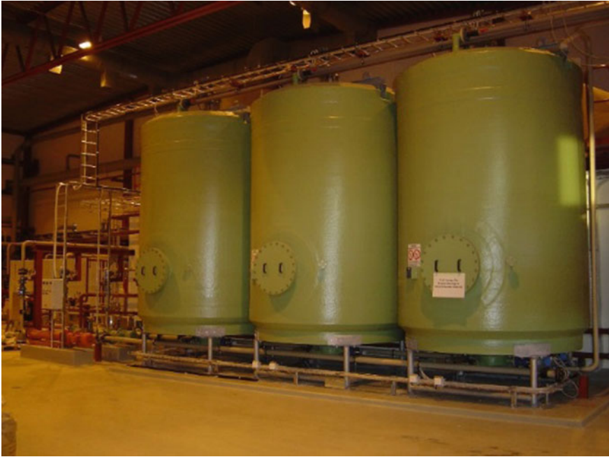
Fig. 5.10 Continuous food waste pasteurization system
