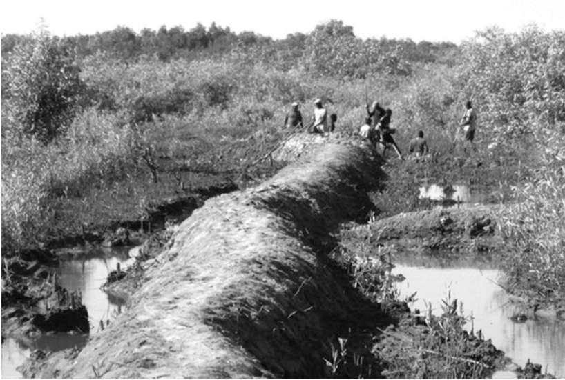
Fig. 2.2 Men building new dike
